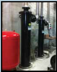
Cleaning chilled water, Axima Belgium
